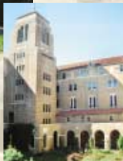
The main building and the inner court
